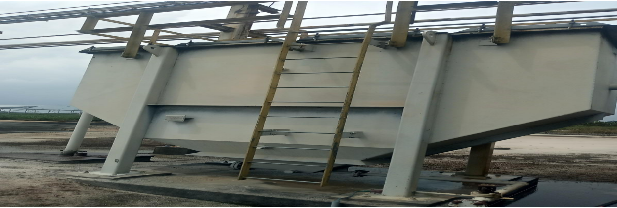
Sludge Containment Pond 1
